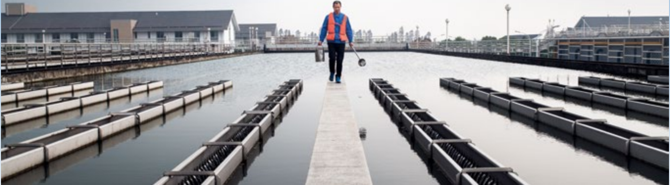
Wu Junhui, Chief of Operations at the Haiyan plant, takes a water sample back to the lab for testing.
